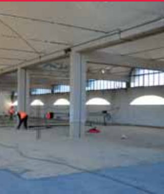
Seismic Upgrade of Prato, Italy
