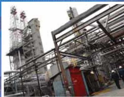
Structural Strengthening and Seismic Upgrade of Valero Refinery Coker Wilmington, USA.
