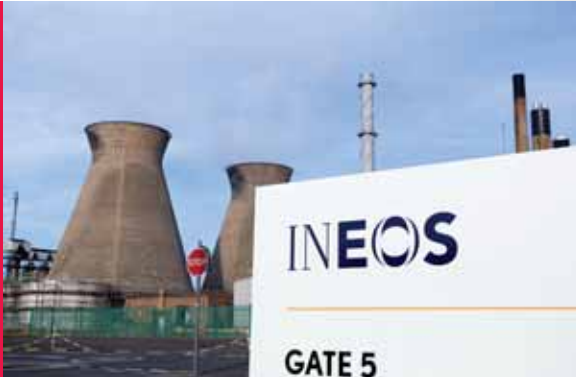
Structural Repair and Protection of steel support columns of INEOS Enterprises, Salt Plant, UK
