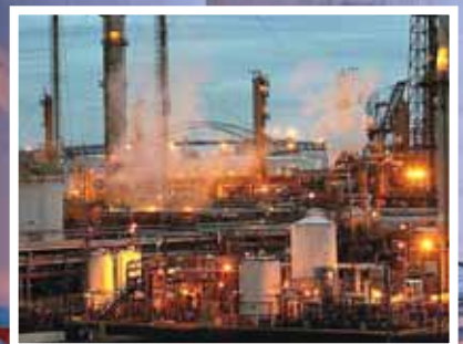
Structural Strengthening of Terminal island Wastewater treatment Plant , San Pedro, USA.
