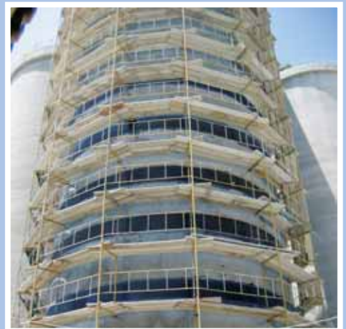
Pre-stressed Concrete Pipe Repair of PPL Montana, USA
