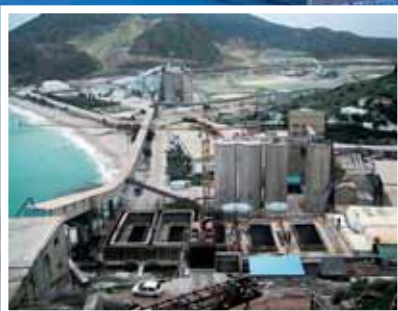
Structural Repair and Strengthening of four-silo Perite complex of S&B Industrial Minerals , Milos, Greece.
