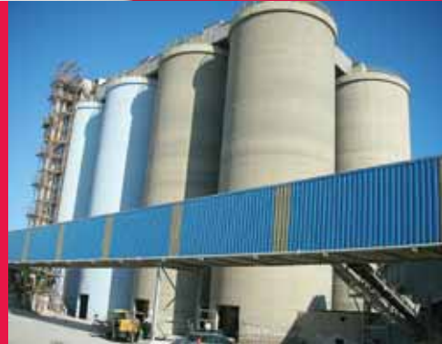
Structural Strengthening Perilite silo of S&B Industrial Mineals, Milos, Greece
